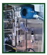
Single Line Panels provide all the necessary sample conditioning components to prepare 50 to 2500psi boiler water samples for analysis.
